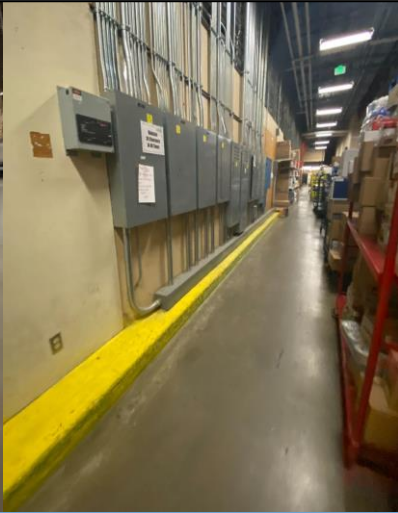
Electrical panels in backrooms:
