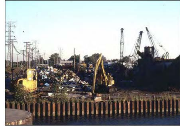
68. Illinois Scrap Processing, view from river, November 1990
