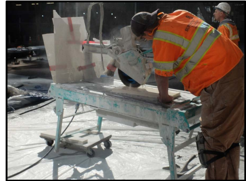
Worker wet-cutting a piece of stone
