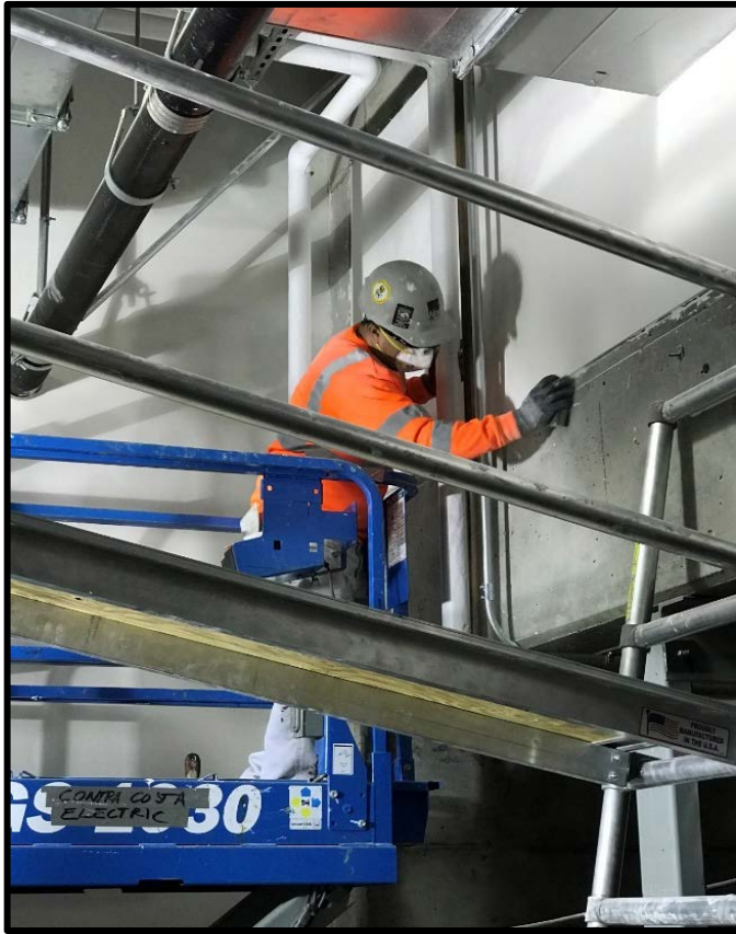
Laborer sanding drywall wearing a respirator
