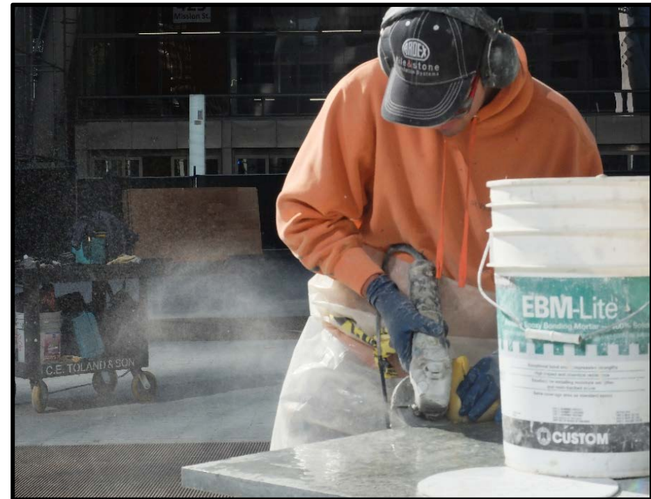
Worker cutting stone that creates respirable silica dust
